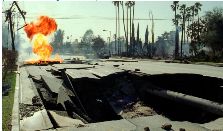
Photo: Northridge Earthquake Damage 1994 (Source: Los Angeles Times)
