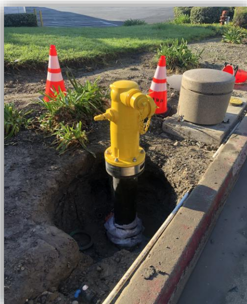
3900 Valley Blvd.– Fire Hydrant Replacement
