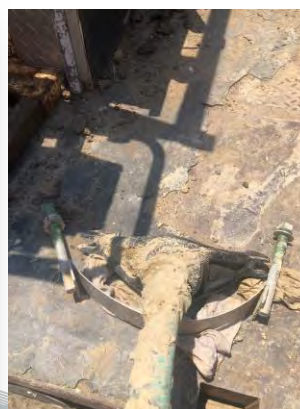
20731 Buckskin Dr. – Service Line and Saddle Replacement
