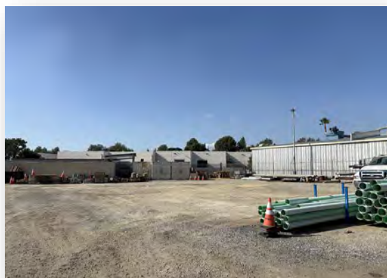
Cleared Pipe Yard to Make Room for Construction
