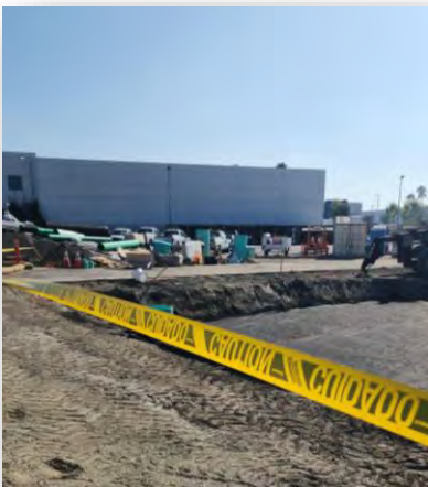
Chamber #2 Installed at the yard
