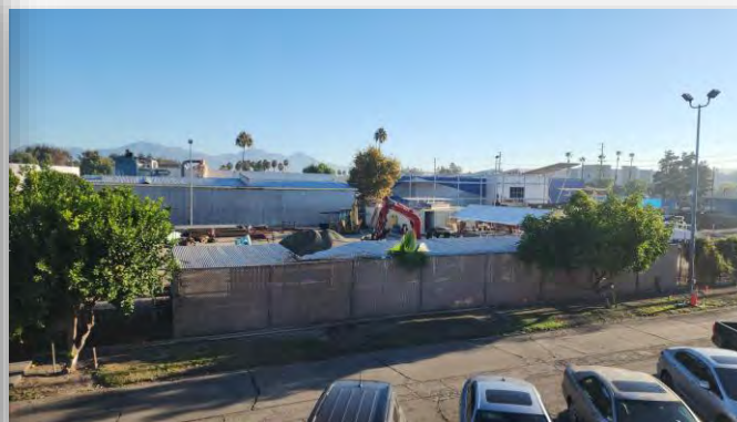
Removing Cages in Pipe Yard for Sitework
