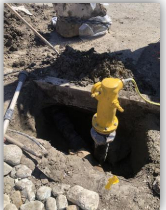
19545 San Jose Ave. - Fire Hydrant Lateral Replacement
