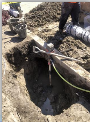
19545 San Jose Ave. - Fire Hydrant Lateral Replacement
