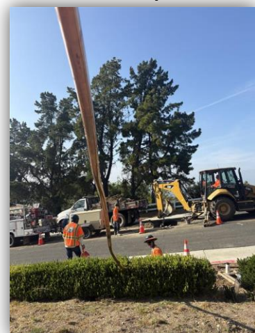
23908 Ridgeline Rd. Service Line Replacement
