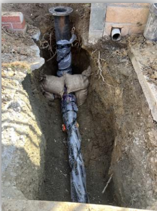
2051 Bing Ct. Blow Off Lateral Replacement
