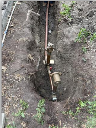
19545 San Jose Ave. - Fire Hydrant Lateral Replacement
