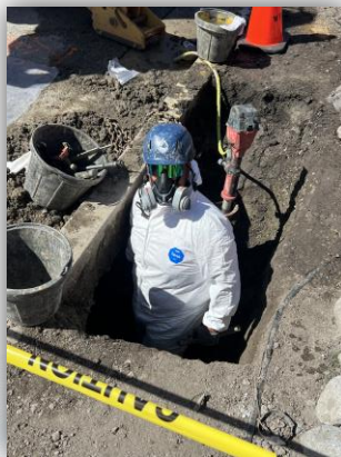
19545 San Jose Ave. - Fire Hydrant Lateral Replacement
