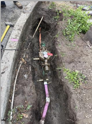
2051 Bing Ct. Blow Off Lateral Replacement
