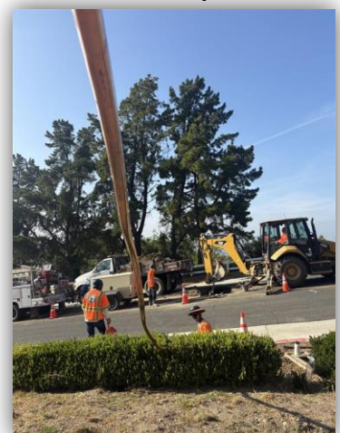
23908 Ridgeline Rd. Service Line Replacement
