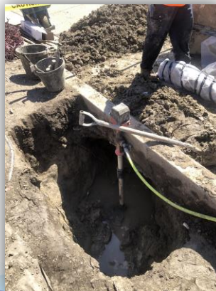
19545 San Jose Ave. - Fire Hydrant Lateral Replacement
