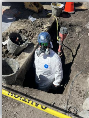
19545 San Jose Ave. - Fire Hydrant Lateral Replacement
