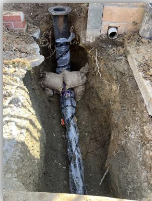
Blow Off Lateral Replacement
