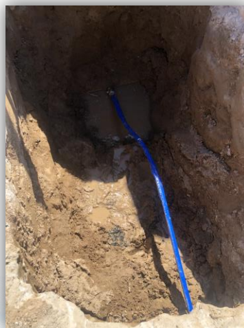
19539 Gravina St. – Service Line Replacement
