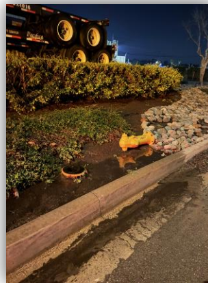
19690 San Jose Ave. Sheared/Replaced Fire Hydrant
