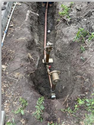
19545 San Jose Ave. - Fire Hydrant Lateral Replacement
