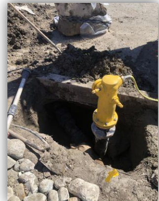
19545 San Jose Ave. - Fire Hydrant Lateral Replacement
