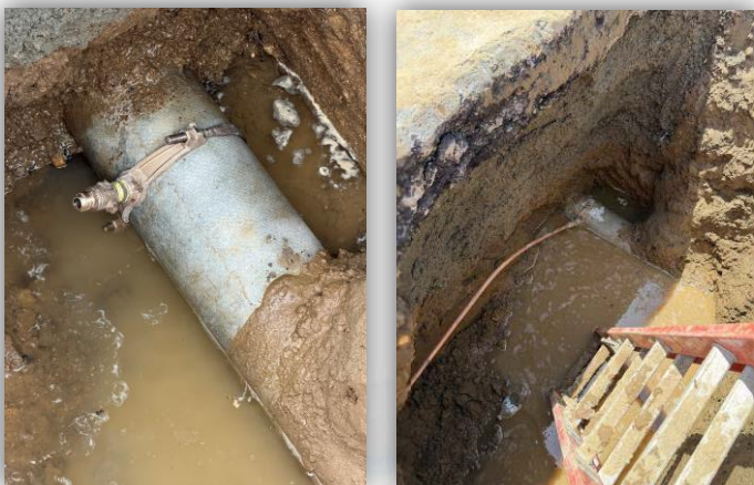
1310 Rolling Knoll Rd. - Service Line Replacement
